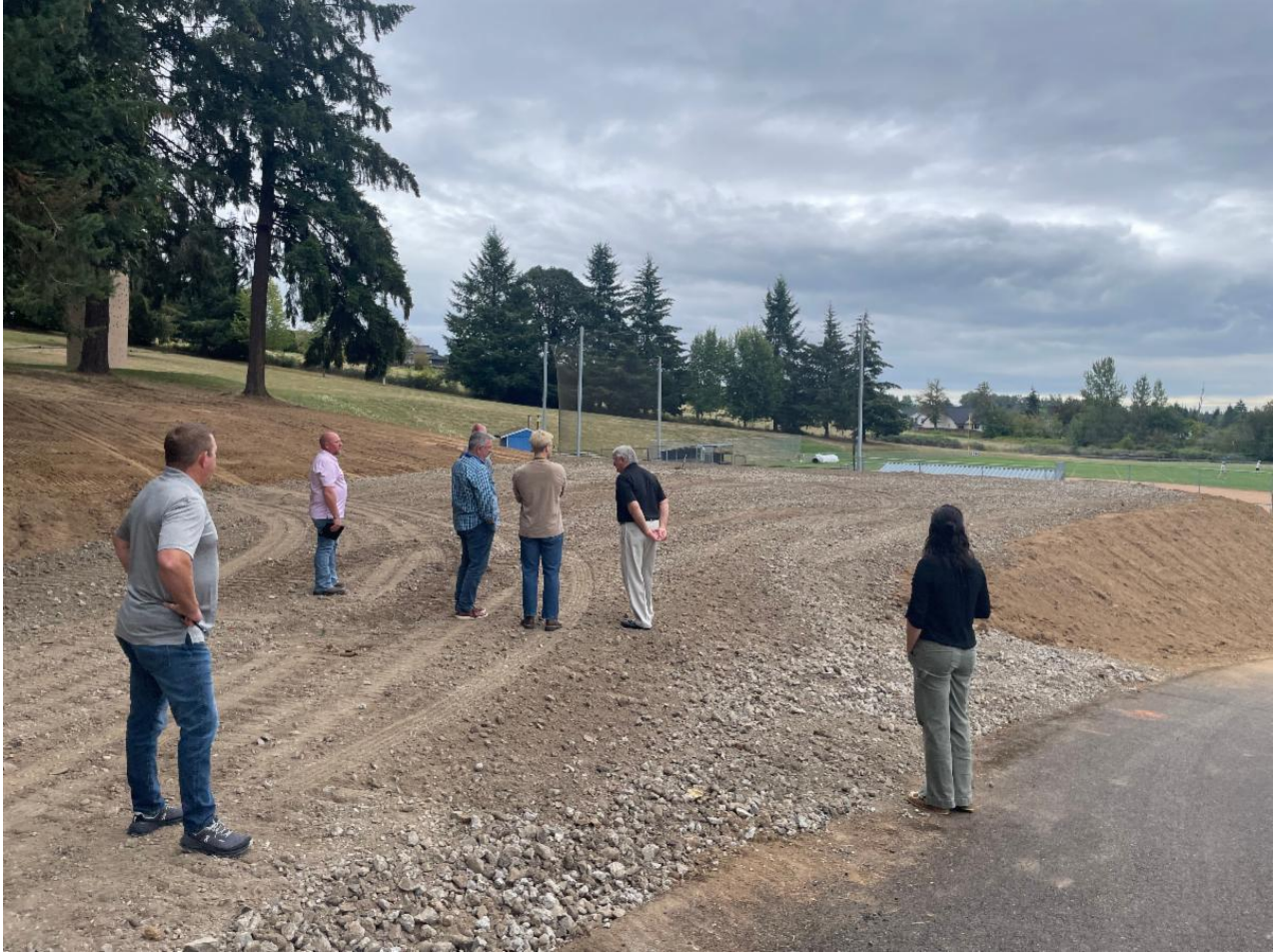
Site prep meeting for the La Center Skilled Trade Building.
