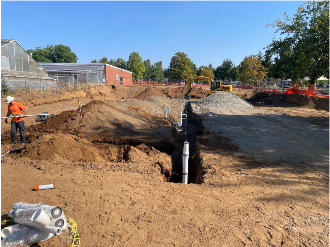
Site work underway at Hudson Bay.
